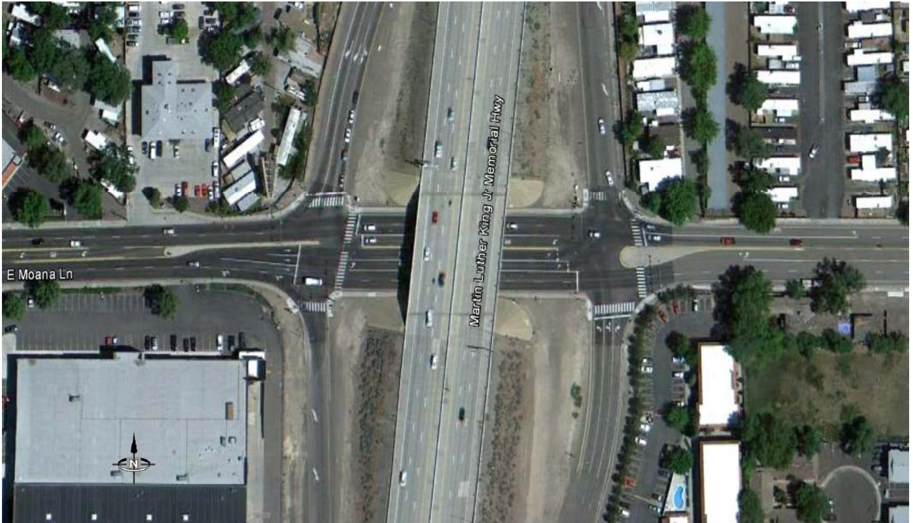
Existing - Moana Lane and I-580 Interchange
