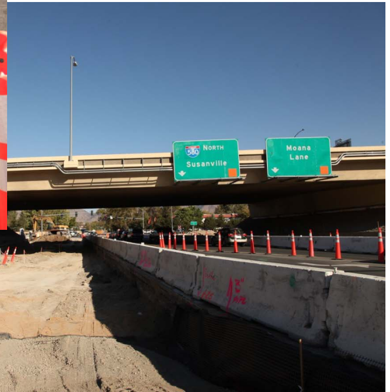
Phase 1 (Soil Nail Walls & Southbound Off Ramp)
