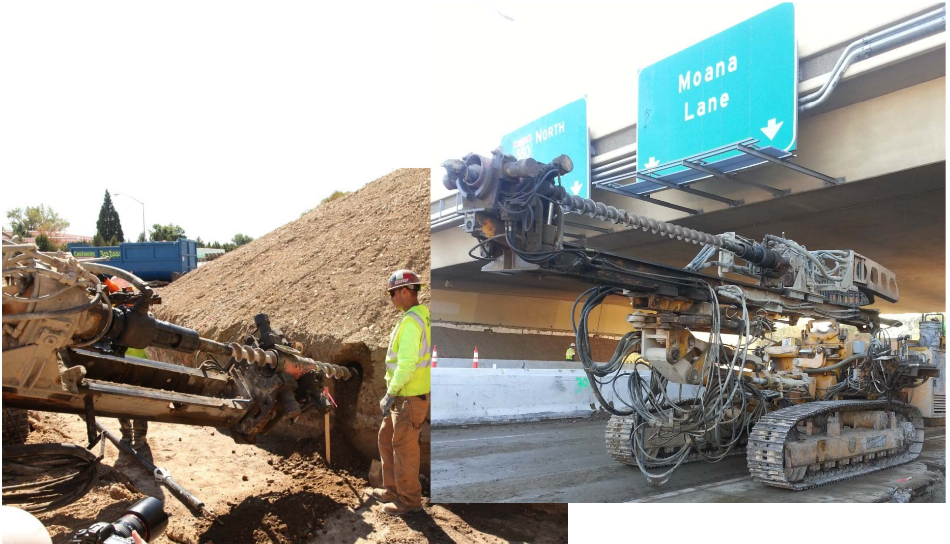
Phase 1 (Soil Nail Walls & Southbound Off Ramp)
