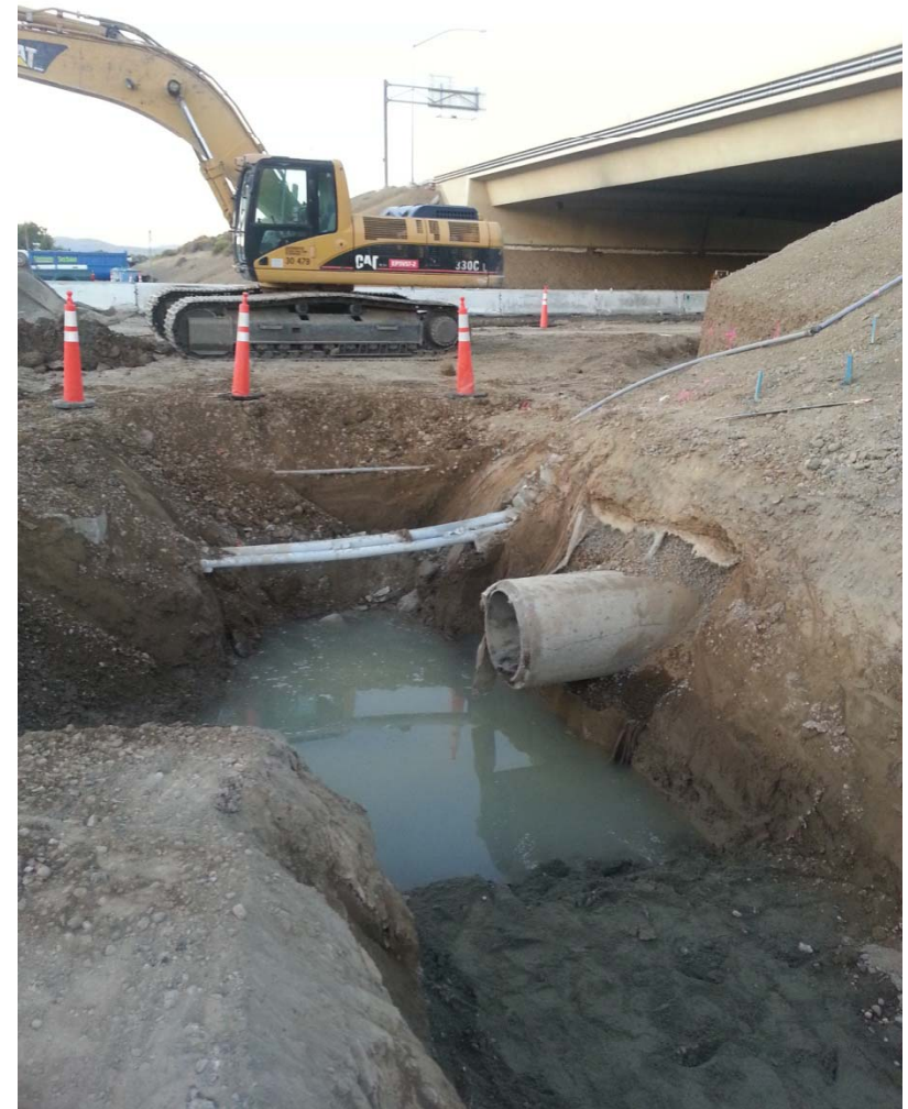
High Groundwater Conditions
